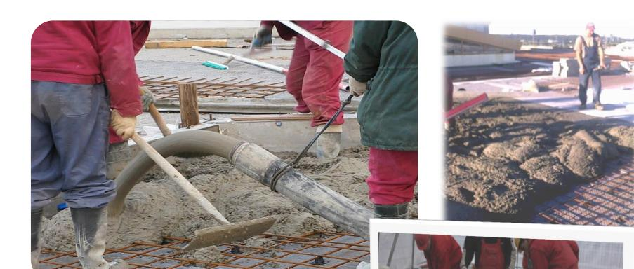
PATCHCONCRETE with W/C = .44 is unloading from the mixer through the house ⊘15 cm or 6" and length at 30 m or 100'. Perfect pumpability of the batch benefited in twice shorter construction time without curing and covering by plastic film also.
