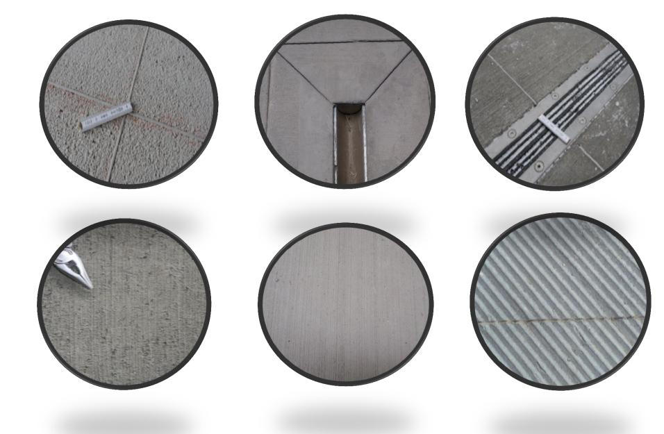
Types of PATHCONCRETE textures for resurfacing of old concrete.
