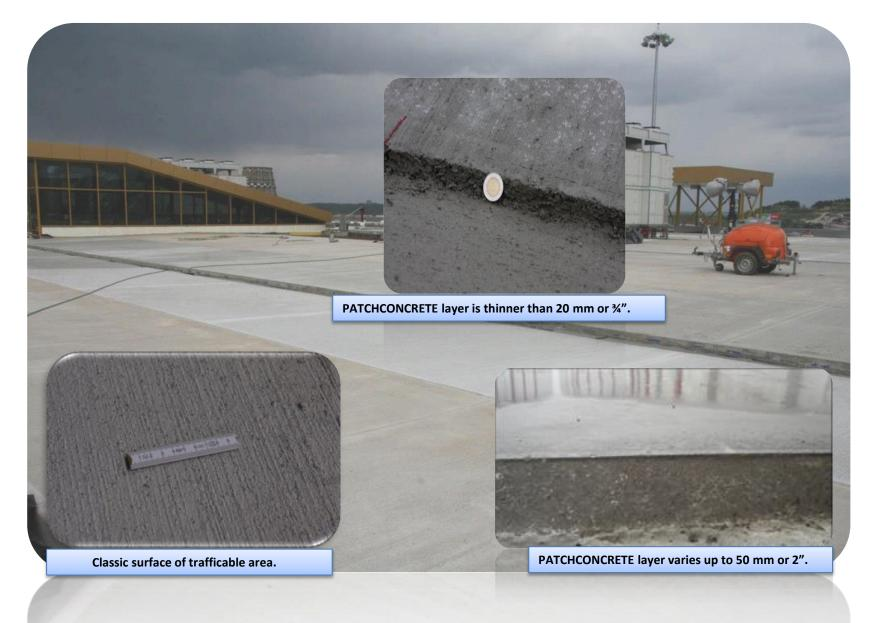
Multiple techniques of PATCHCONCRETE applications resulted in the layers thinner than 20 mm or 3/4" and as thick as 50 mm or 2".
